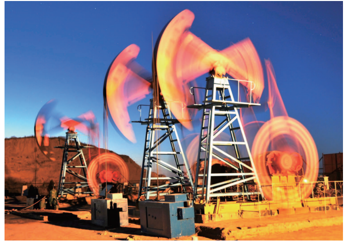
CNOOC Uganda Kingfisher oil field facility project
