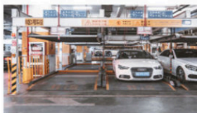
Parking lot Management
