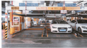
Parking lot Management
