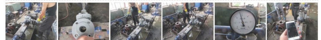
Open/close valve 5times | Open/close valve 5times | Fixed the valve | Beginning test | Set 2.4Mpa | Keep 60s
