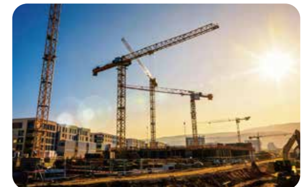
Construction Tower Crane
