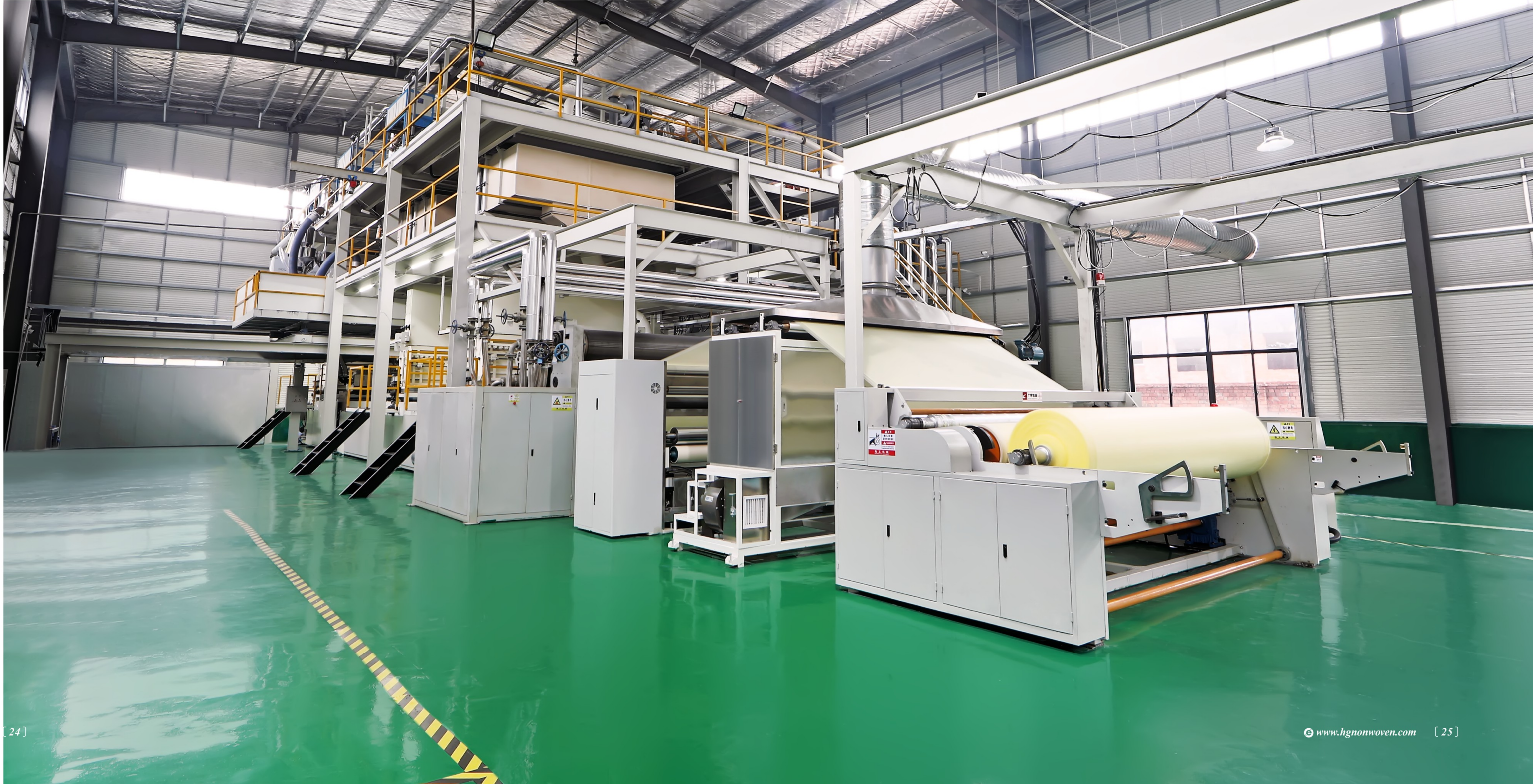
SMMS 丙纶纺粘熔喷无纺布生产线 Polypropylene spunbond and meltblown nonwoven fabric production line (SMMS)
