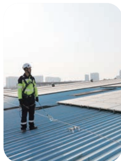
Factory Building Roof
