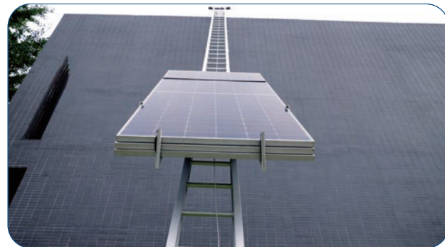
Plant Roof Photovoltaic Installation
