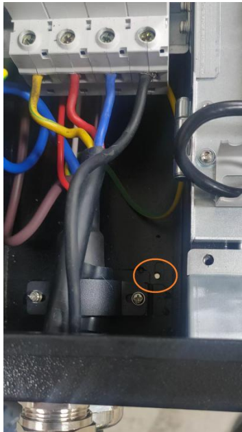
Figure 3. 1. 1-3 Anti-theft screw fixed
