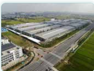
Intelligent inspection in industrial parks
