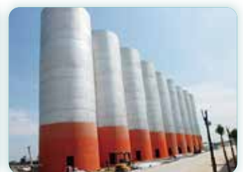
Intelligent inspection in petrochemical tank farms
